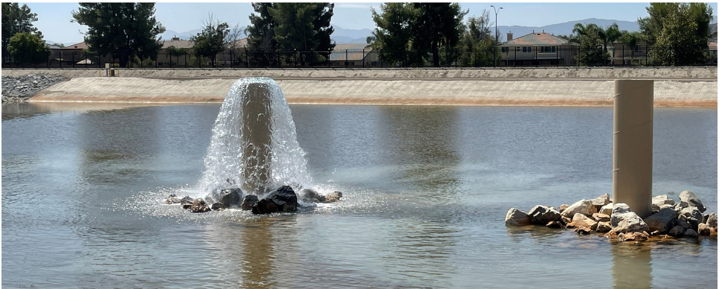
Mountain Avenue West Groundwater Replenishment Basins
