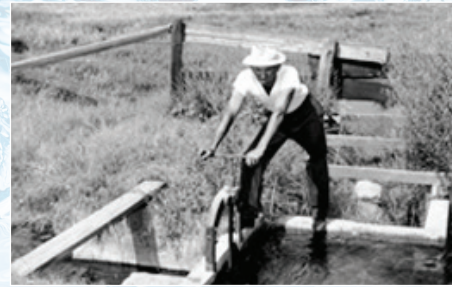
1953 - Colorado River water being turned on at the EMWD ranch
