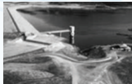
1970s - Filling Lake Perris to bring northern California water to the region.
