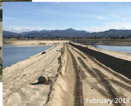
Repairs in the channel from erosion at IRRP North
