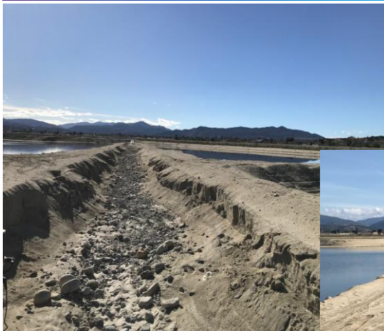
Repairs in the channel from erosion at IRRP North
