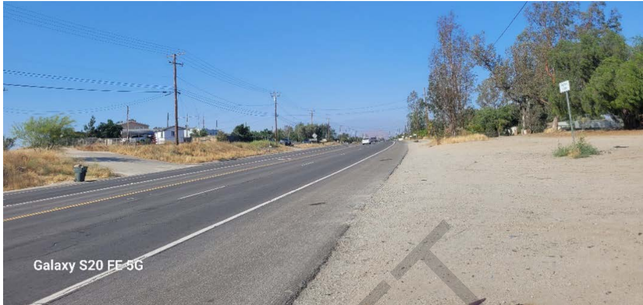
Photo No. 3: Hwy 74, view towards northeast.
