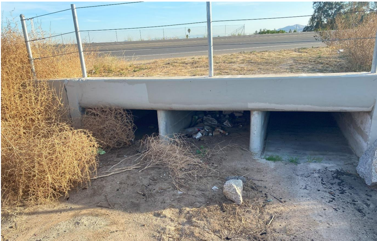
Photograph 12. Triple box culvert along Highway 74, facing west. December 8, 2023.
