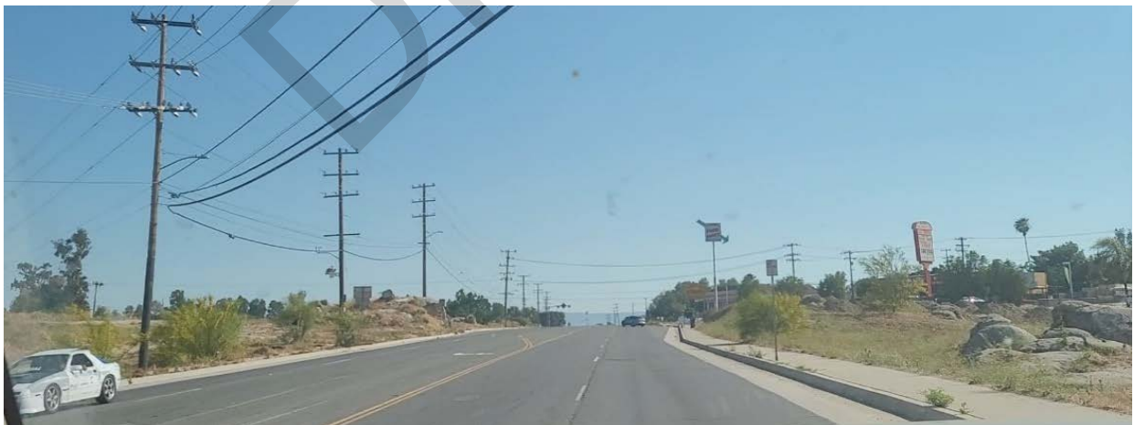
Photo No. 2: Hwy. 74, view towards southwest.
