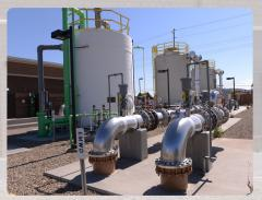
Where Does The Salt Go?: At the end of the reverse osmosis process, the salty brine is discharged into the Inland Empire Brine Line. It is sent through the 70-mile pipeline to a treatment plant on the coast in Orange County, where it is ultimately discharged into the ocean.
