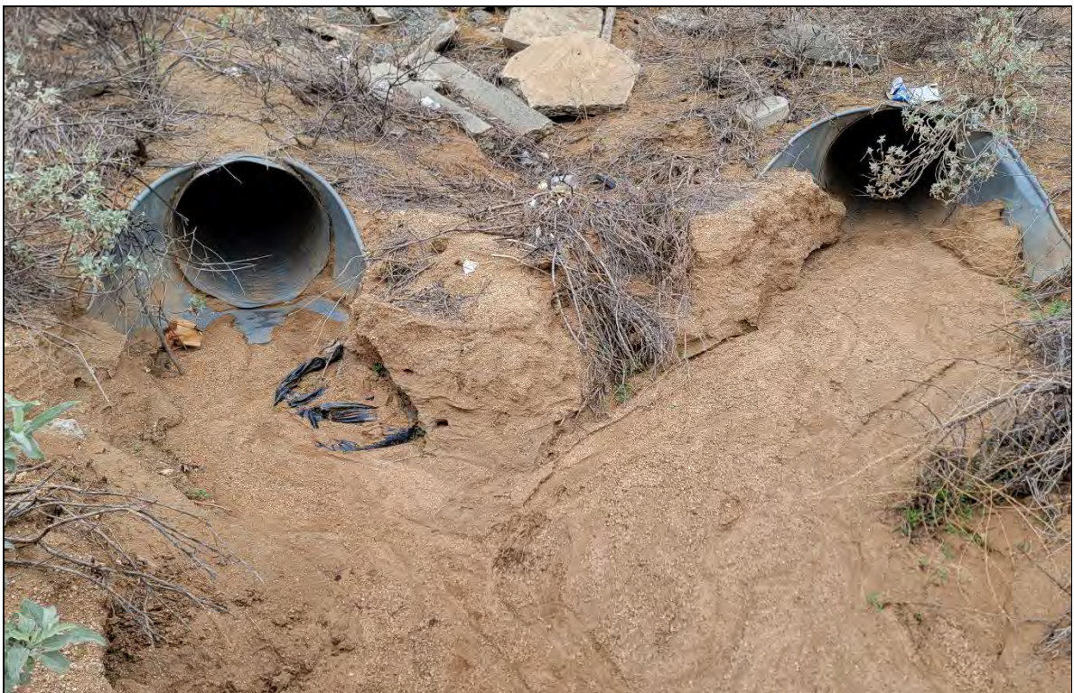
Photograph 20: View upstream towards two 30" culverts for EF2 (left) and EF3 (right), facing west, and their confluence just east of Moreno Beach Drive. Channel continues as a single ephemeral channel downstream conveying flows to the east.
