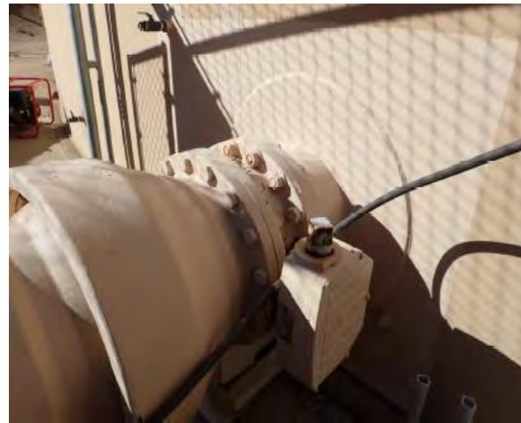
Figure 18: Inlet/outlet penetration in good condition
