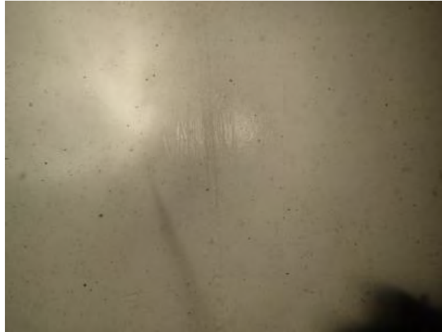
Figure 3: Tank interior shell wall with few isolated corrosion spots.
