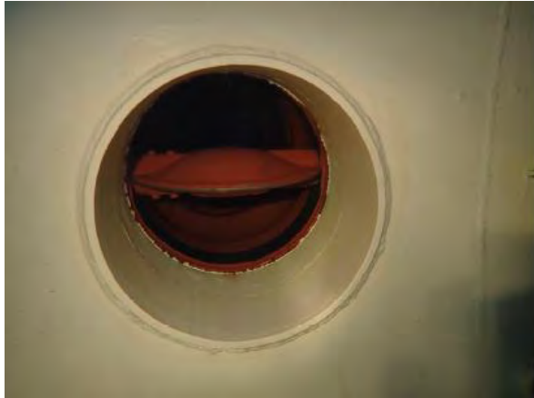
Figure 6: Inlet/outlet penetration with no corrosion
