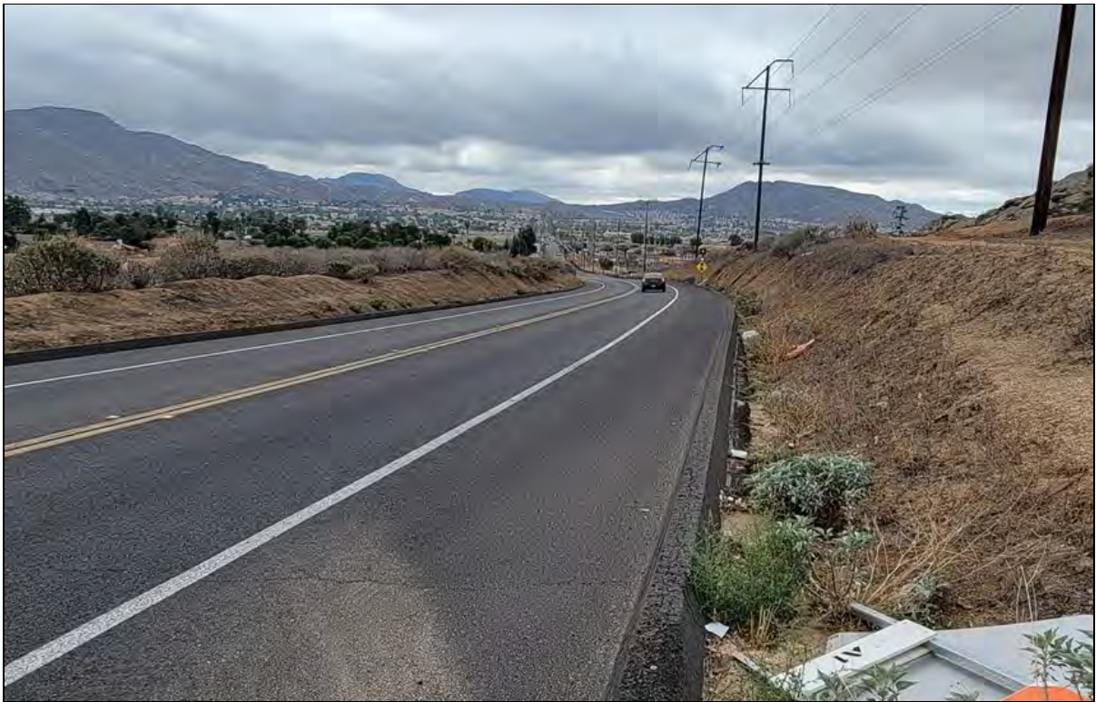
Photograph 7: View of Moreno Beach Drive and proposed Transmission Pipeline location, facing south from driveway at 13325 Moreno Beach Drive.
