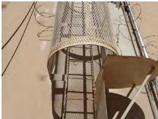
Figure 22: Exterior ladder in overall good condition with minor corrosion spots
