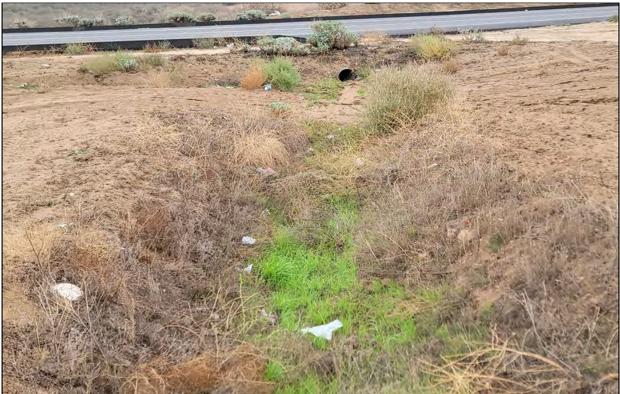
Photograph 10: View of erosional feature EF1, facing downstream and southeast towards its intersection with a metal culvert beneath Moreno Beach Drive.
