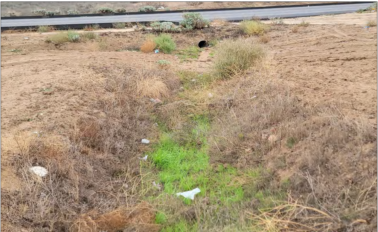
Photograph 2: View of Drainage 1, facing downstream and southeast towards its intersection with a metal culvert beneath Moreno Beach Drive.
