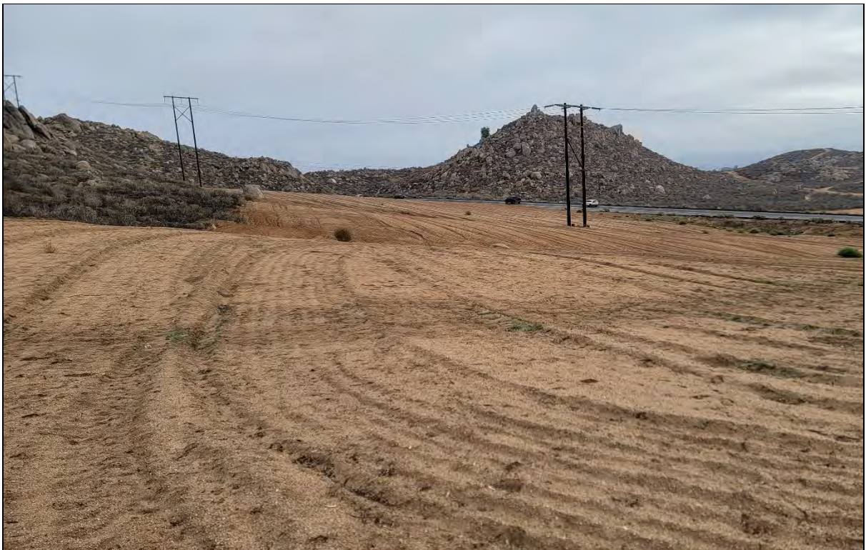
Photograph 4: View of Phase 1 water storage tank location facing northeast from southwest boundary of proposed water tank location. Photo depicts disturbed land north of existing Pettit water storage tank.
