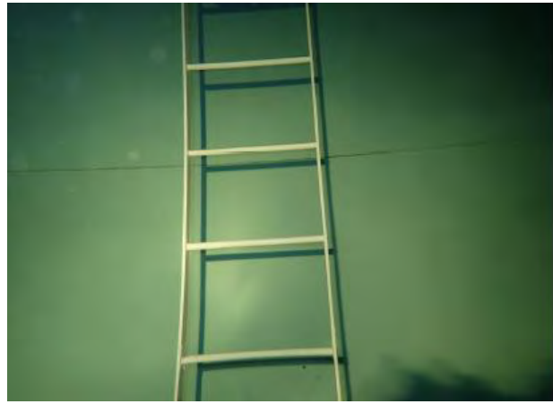
Figure 12: Interior ladder in good condition
