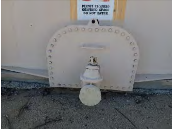
Figure 20: Doghouse drain in overall good condition
