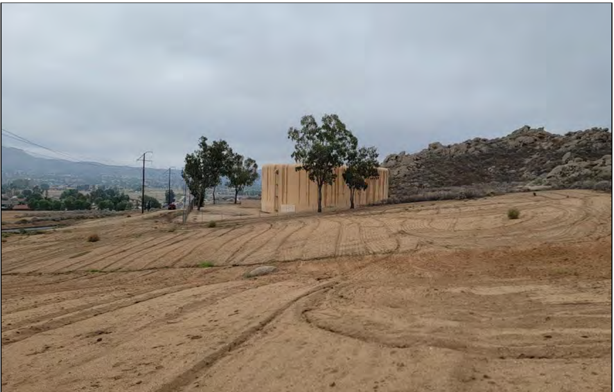
Photograph 6: View of Phase 1 water storage tank location, facing south from northern boundary of proposed grading limits. Photo depicts disturbed land north of the existing Pettit Water Storage Tank and brittle bush scrub west and south of the existing Pettit Water Storage Tank.
