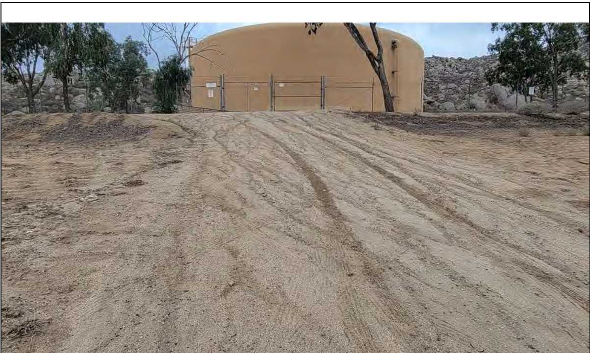
Photograph 1: View of east side of existing Pettit Water Storage Tank and entry gate, facing west. Photo depicts unpaved driveway and location of proposed transmission pipeline.
