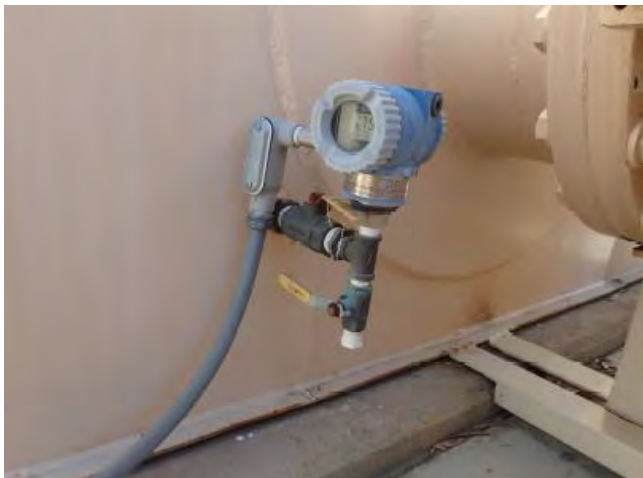
Figure 17: Penetration for level indicator in good condition with no visible corrosion
