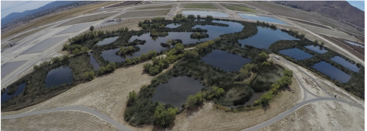
EMWD's Wetlands at the San Jacinto Valley Regional Water Reclamation Facility
