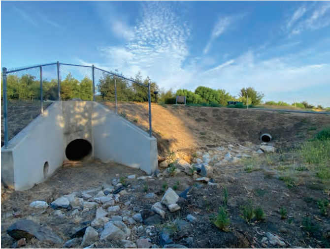
Photo 5: View looking northeast at Drainage C located along the eastern side of Washington Street.
