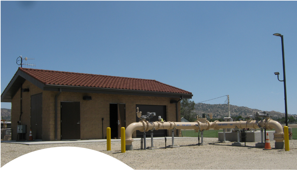
Completed well building
